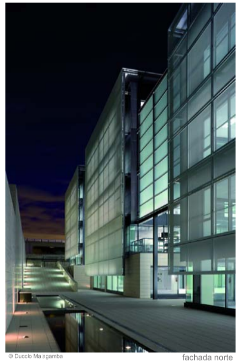
fachada norte north facade view
