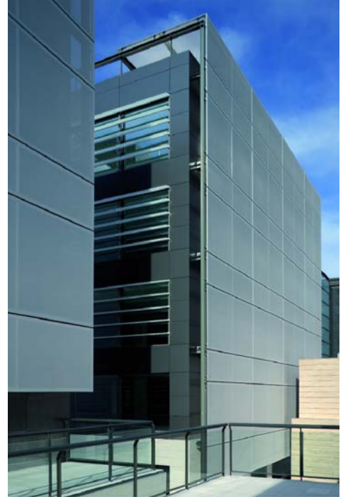
fachada sur_unión entre bloques south facade_cladding between blocks
